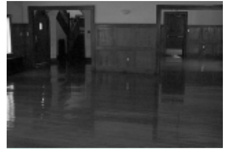
Main level floors received another coat of Polyurethane, the third in three years, which should ensure that the hard wood is adequately protected.
